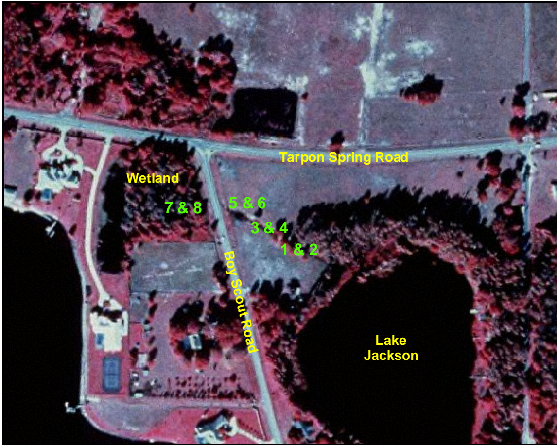
Figure 7. Outlet conveyance system for Lake Jackson in Hillsborough County, Florida.
